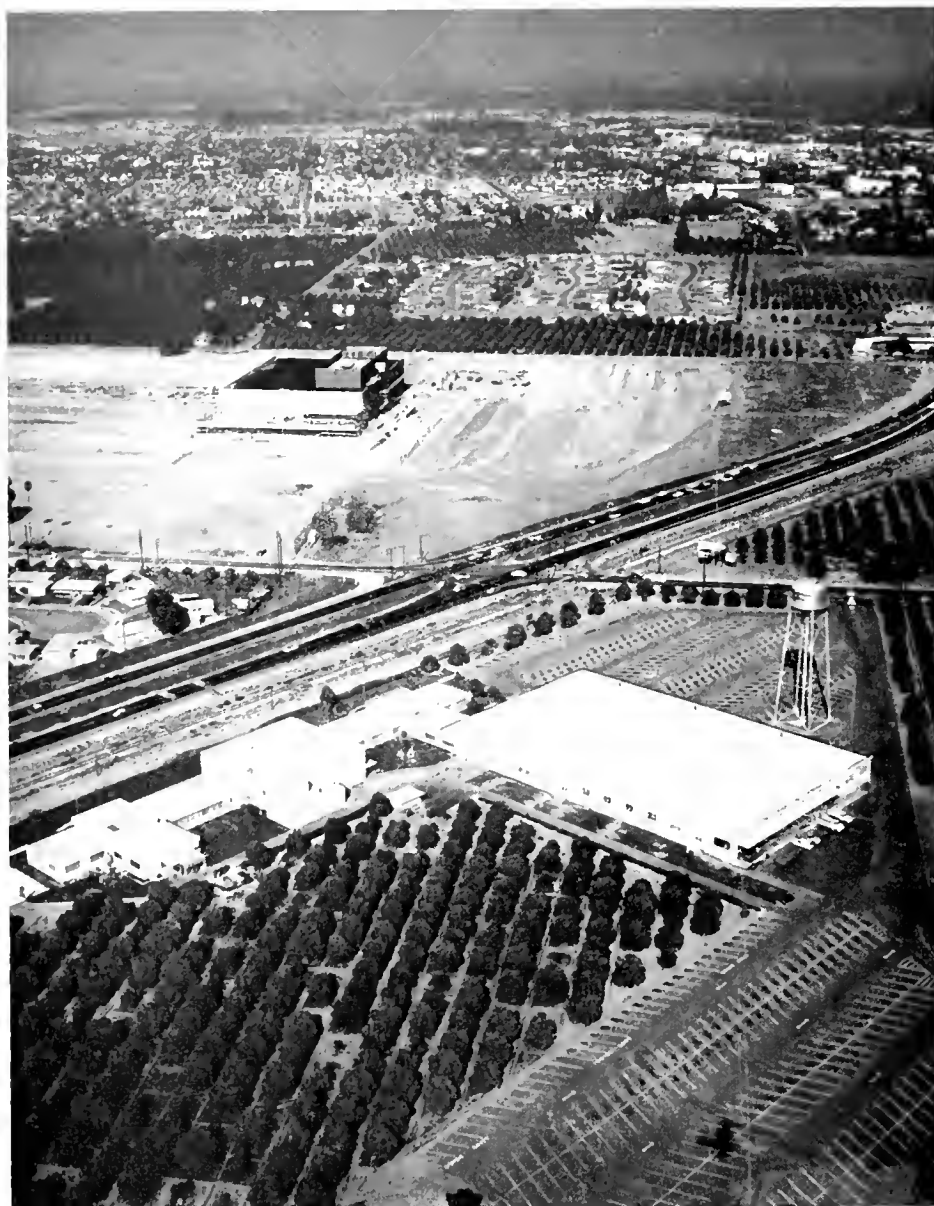
Looking easterly showing, center left, new Broadway-Anaheim Shopping Center under construction in City of Anaheim, with extensive parking space provided for shoppers adjoining the Santa Ana Freeway. In foreground is shown manufacturing plant of Robertshaw Fulton Controls Company, with adequate parking space provided convenient to buildings.
